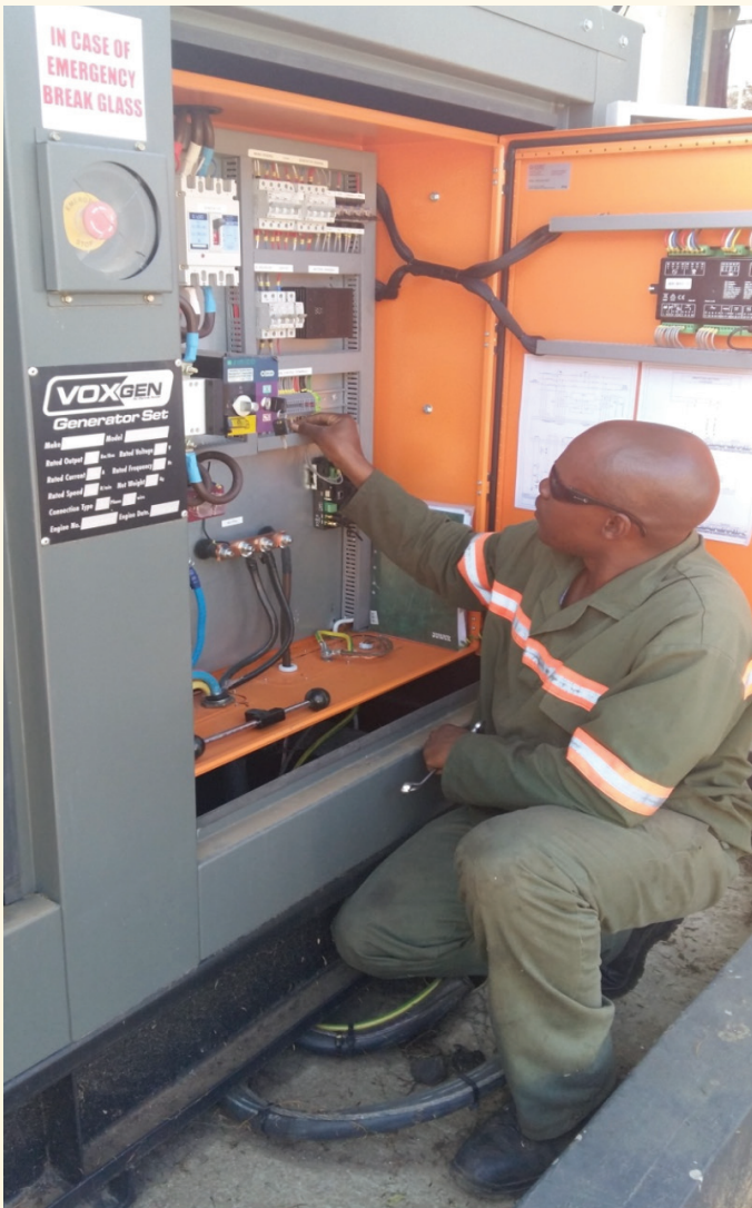
A police engineer attending to faults
